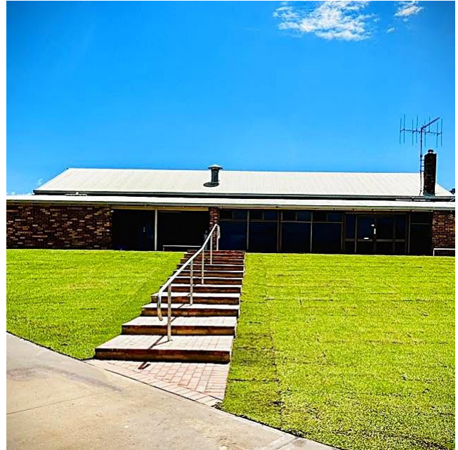
Broomehill Recreation Complex
