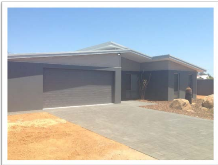
Great Southern Housing Initiative Lot 8 Taylor Street, Tambellup completed
