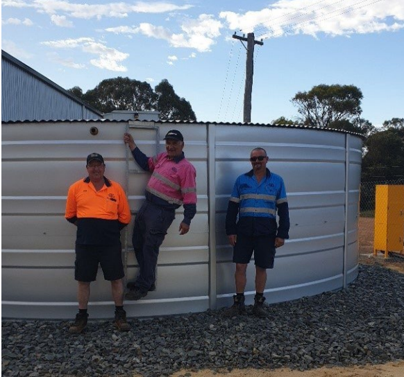
New tank installed, Tambellup Depot
