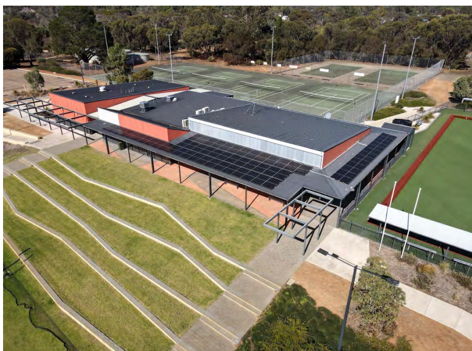
Tambellup Community Pavilion – Solar Panels
