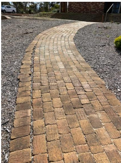
1. Broomehill Recreational Complex carpark/oval access - before
