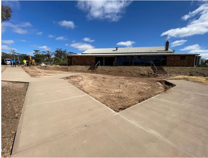
3. Broomehill Recreational Complex carpark/oval access – after
