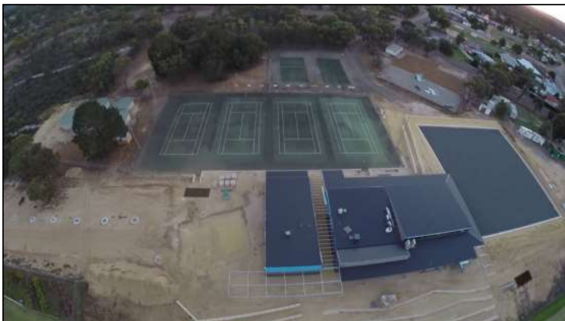
Tambellup Community Pavilion progress – April 2017
