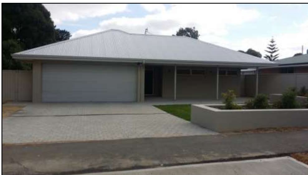
Construction of Executive Residence – 2016
