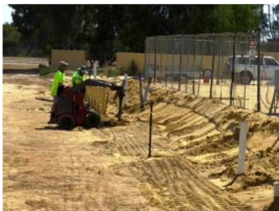
Building the retaining wall
