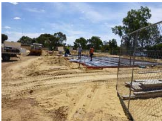
Preparing to lay the slab for Unit 6
