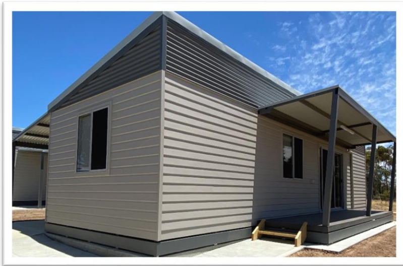
Great Southern Housing Initiative Broomehill Caravan Park
