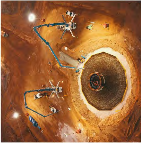
Concrete pour of a wind turbine foundation underway.
