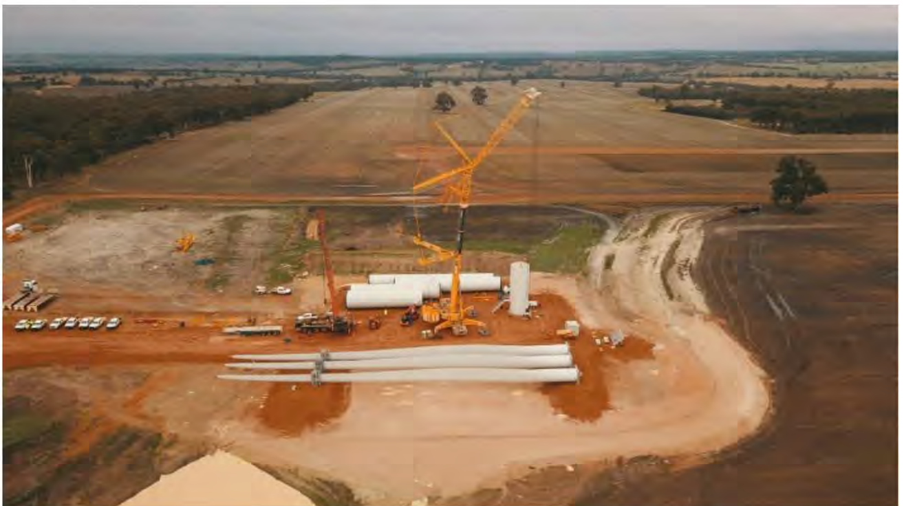
Installation of a tower underway at Flat Rocks Wind Farm Stage 1
