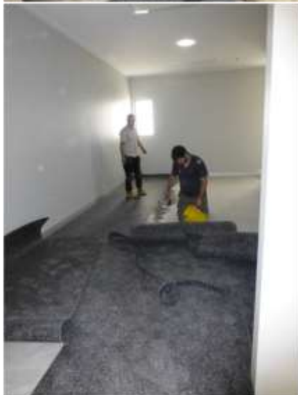
Left Laying rubber floor covering in the changerooms
