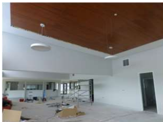
Acoustic timber ceiling in the main hall
