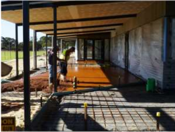
Concreting of verandahs
