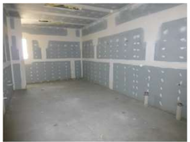
'Wet' area of changeroom 1
