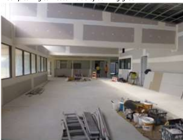
The main hall (minus acoustic timber ceiling lining)
