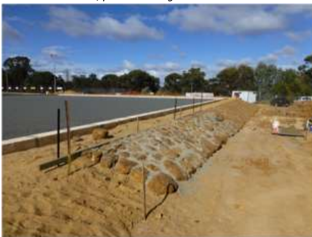
Rock pitching to western side of bowling green
