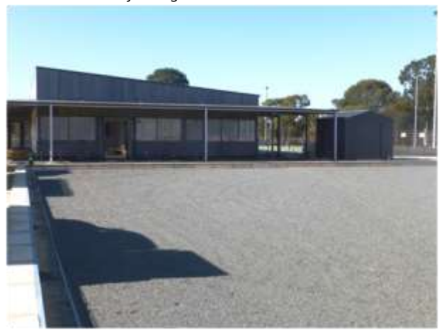
Bowling Green shed
