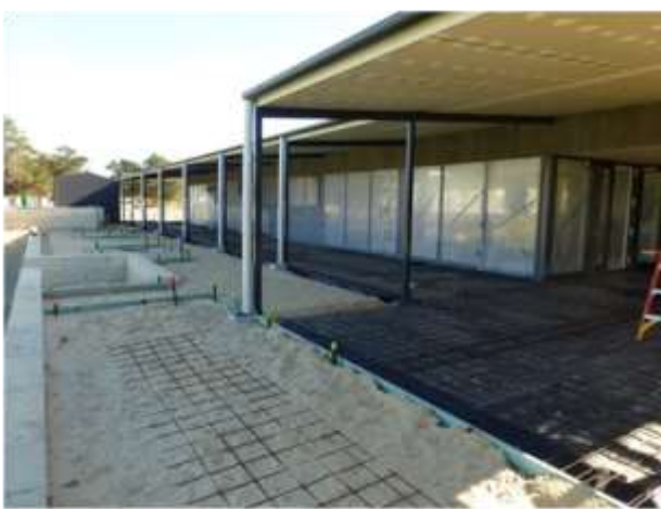
Tennis court side, pre concreting
