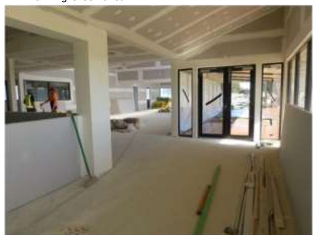
The main hall from the kitchen servery
